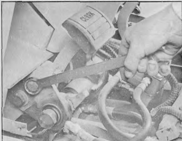
Plate 9842. Torque Outboard Bearing Bolts
